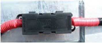
Tippa main fuse 150A is located in close proximity of vehicle battery
