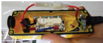
Control fuse (5A glass type) located within pendant control
